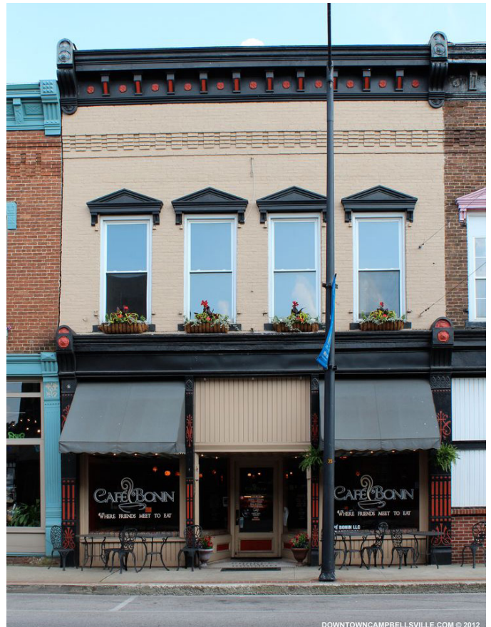
Storefront Renovation in Campbellsville, KY
