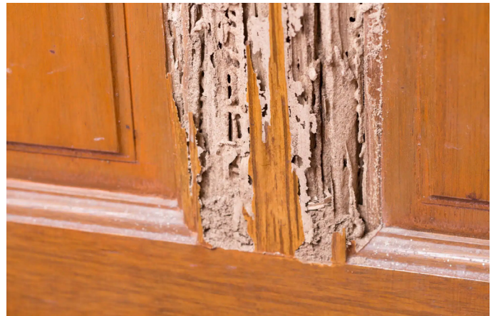
^ Termite damage
