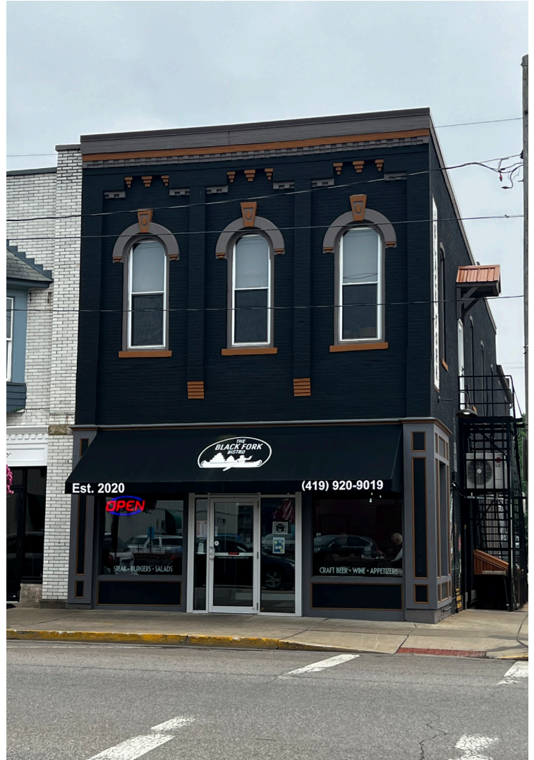
^ The Black Fork Bistro Building Renovation
