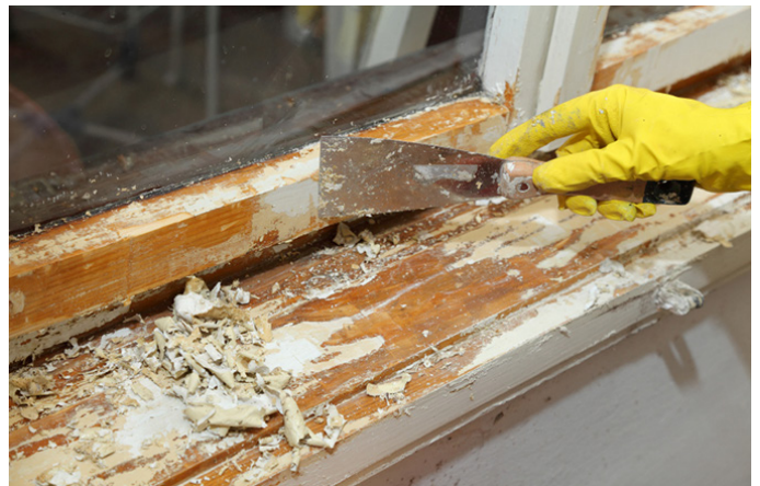
▲ Removing old window paint with a scraper
