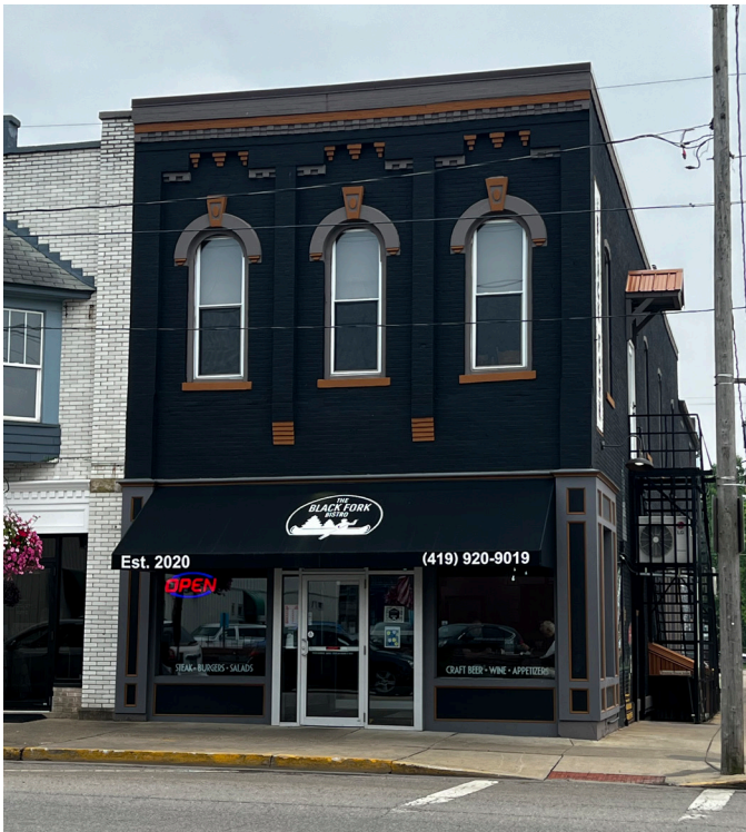
▲ The Black Fork Bistro Building Renovation
