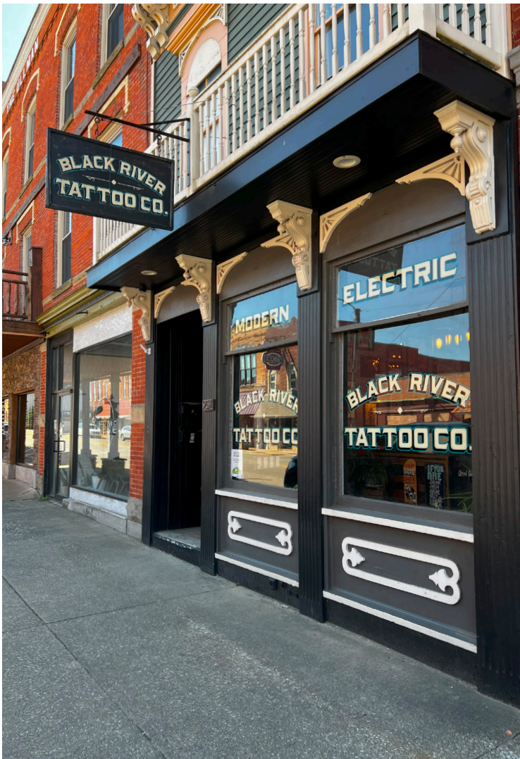
▲ Black River Tattoo Co. Storefront Renovation
